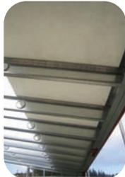
3. While someone is holding the sheet in place, secure each corner with self-tapping screws. This ensures the sheet remains in place while the glue is setting.
